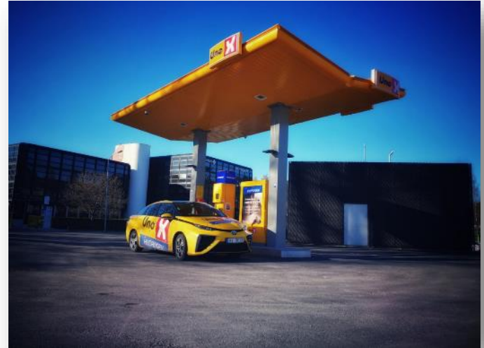
Uno-X Hydrogen fueling station at Kjørbo, Norway Onsite hydrogen production from solar power
