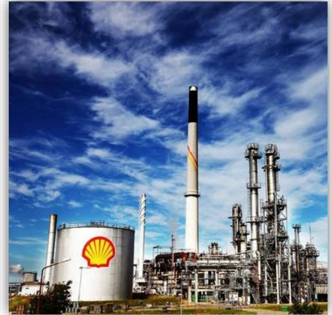
Shell oil refinery in Fredericia, Denmark
