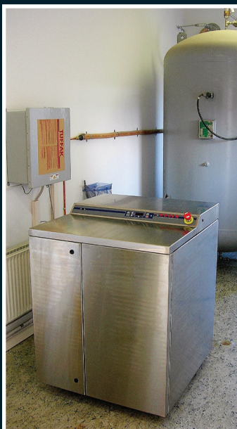
Typical S Series Hydrogen Gas Generator Installation for Upper Air Stations
