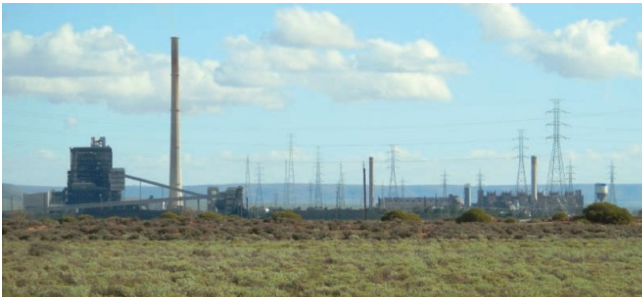
Figure 1. Northern Power Station in Port Augusta switched from bottled hydrogen to an on-site hydrogen generator to supply its two 260MW turbines with cooling gas.
