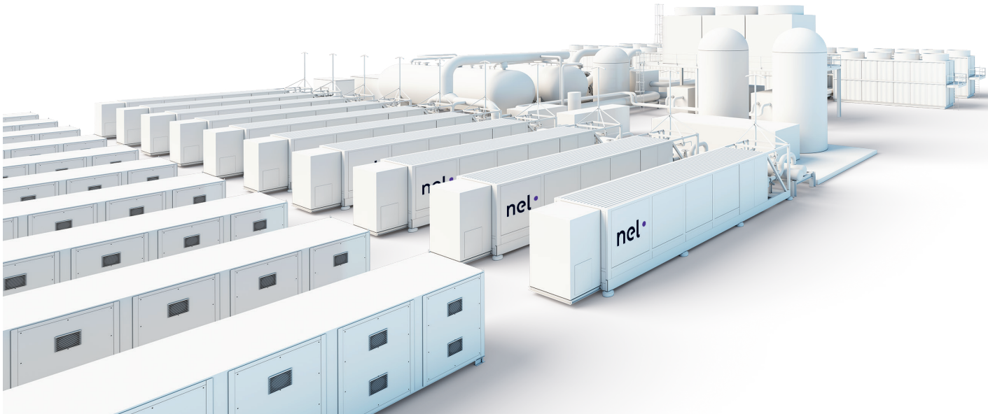
100 MW PEM electrolysis plant featuring ten PSM containerized modules.
