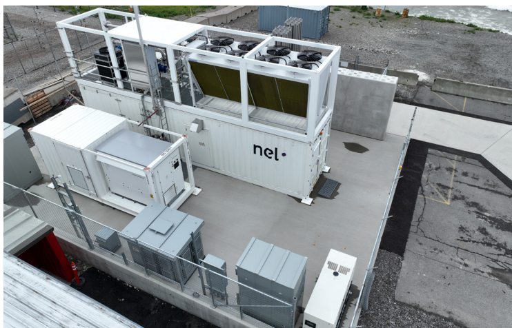
Figure 1. Containerised PEM electrolysers are capable of producing 500 m 3 /h or over 1 tpd of hydrogen.
