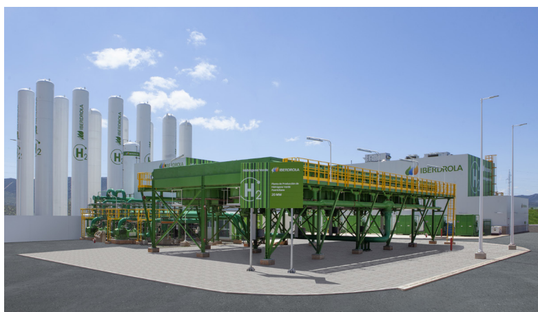
Figure 2. The 20 MW PEM plant at the Iberdrola-Fertiberia facility in Puertollano, Spain, is the largest electrolysis plant currently in operation providing green hydrogen for green ammonia production.
