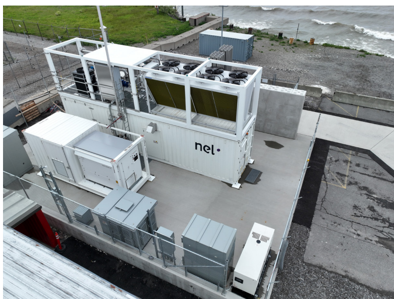
Figure 1. Nel containerised PEM electrolyzers are capable of producing 500 m 3 /h of hydrogen or over 1 tpd. The unit above is located at a Constellation Energy nuclear plant in upstate New York, US.
